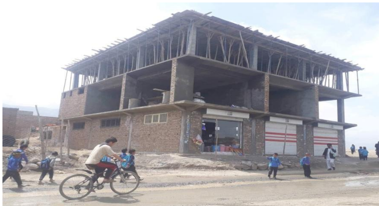
Fig3.2 The original structure
